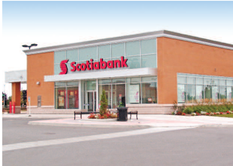
Scotiabank (Richmond Hill, Ontario) HA-8 - Push installations.
