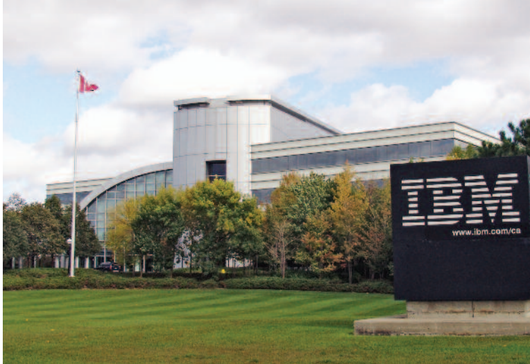
IBM (Markham, Ontario) HA-8 - Centre Spindle installations.
